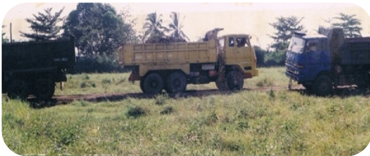
Construction of the road network at CEROS now completed.
