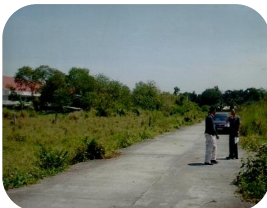
Concrete road inside the subdivision
