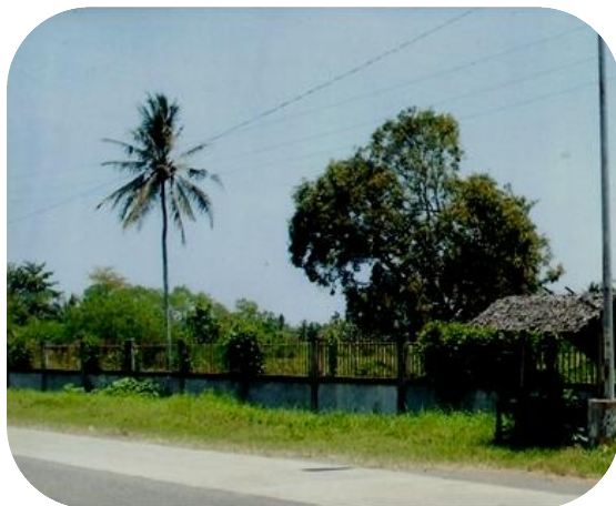
Front View of Ceros enclosed by a concrete fence
