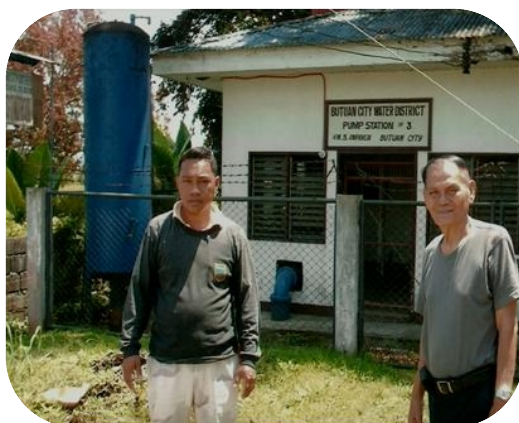
Butuan City Water District Pumping Station adjacent to the subdivision, east side
